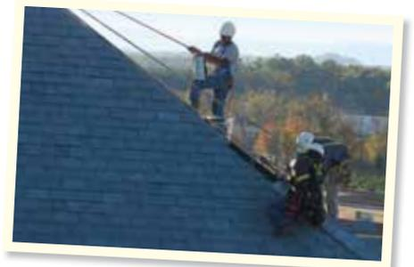
■ Dunn Roofing and Sheet Metal Inc.’s safety plan called for anchor points at the ridge, lifelines, snap hooks, lanyards and full body harnesses, as well as a scaffolding system.
